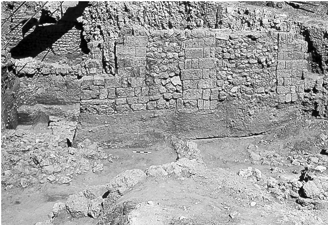
Figure 5.15. W.800 built in ashlars pier alternating with rubble wall technique. Kaplan Archive.
